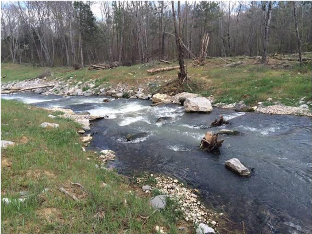
Figure 5. Boulder and Logs in a Constructed Riffle
